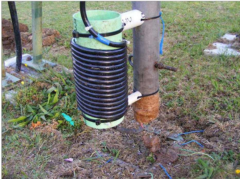
Closeup of the ZL1ALZ "Ugly Balun"
